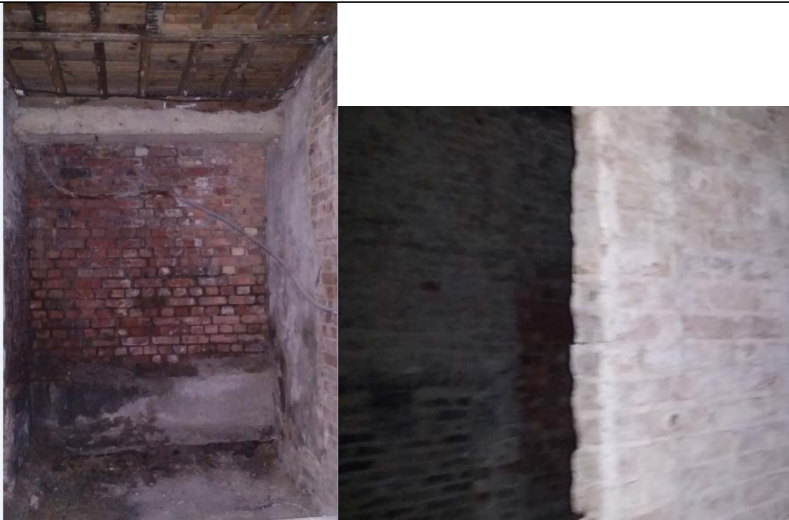
Basement of 32 Blomfield Villas (indicative of the size/state of all the basement spaces to be turned into 3 bedroom flats).
